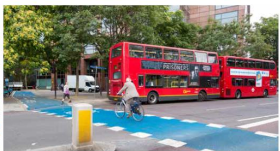
Signal-controlled cycle crossings, using elephant's footprint markings through the junction
