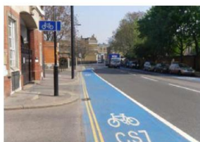
Mandatory cycle lanes, including an example of a sign to diagram 959.1 of TSRGD
