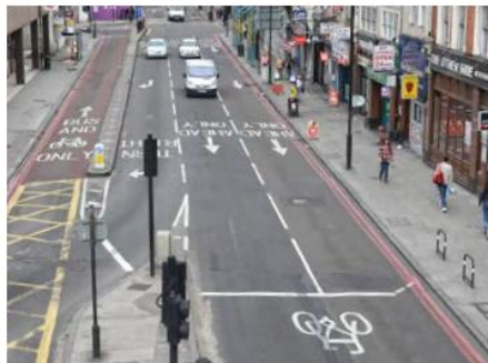
With-flow bus lane (left) and contraflow lane with 'bus and cycle' marking (right)
