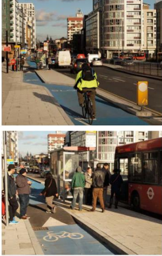
Bus stop bypass at Stratford High Street, showing pedestrian crossing over cycle track
