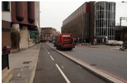
Two-way track at Goodman's Yard, City of London
