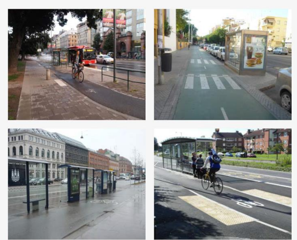
Examples of bus stop bypasses – clockwise from top left: Stockholm, Seville, Brighton & Hove, Copenhagen
