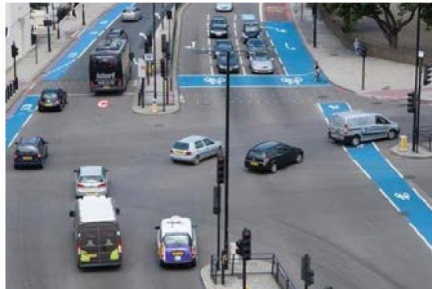
Dashed markings used to show continuity of lanes through junctions
