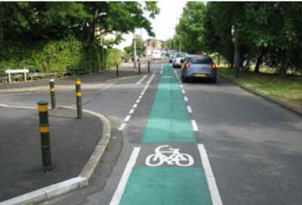
Mandatory lane becomes dashed past side road (lane marked away from kerb and side road)
