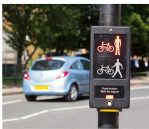
Nearside push-button control for toucan crossing
