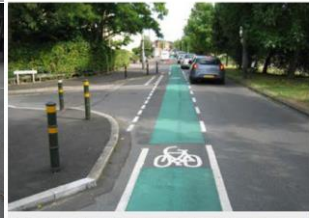
Mandatory lane becomes dashed past side road (lane marked away from kerb and side road)
