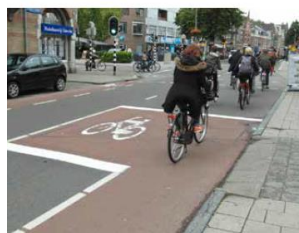
ASLs with lead-in lanes are also used in other countries – as in this example from Utrecht
